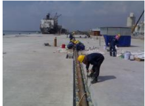
Installers grinding the welds
