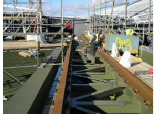
With two rail 'Welding the rails after they had been accurately aligned.'
