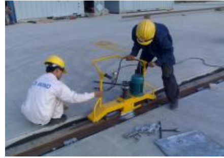
Installers grinding the welds
